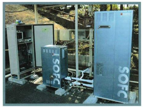
Fig. 1. SOFC-based residential CHP system showing the SOFC unit (left) and the hot water tank (right).
