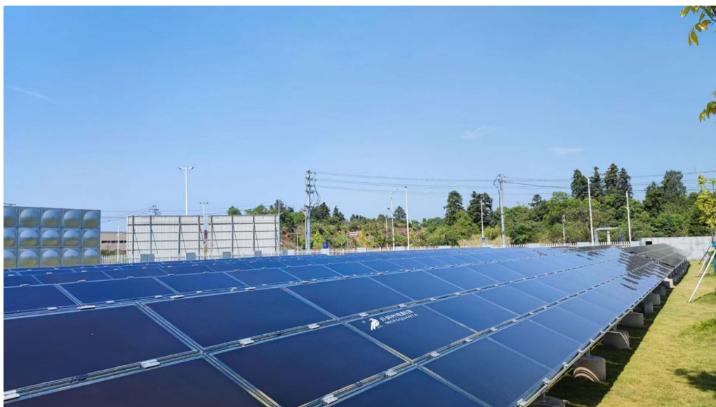
Figure 2. Picture of 100 kW perovskite grid-connected solar farm from Micoquanta.
