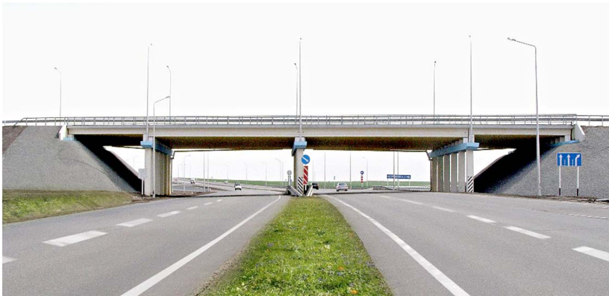
Figure 2. Reinforced concrete overpass with four spans.
