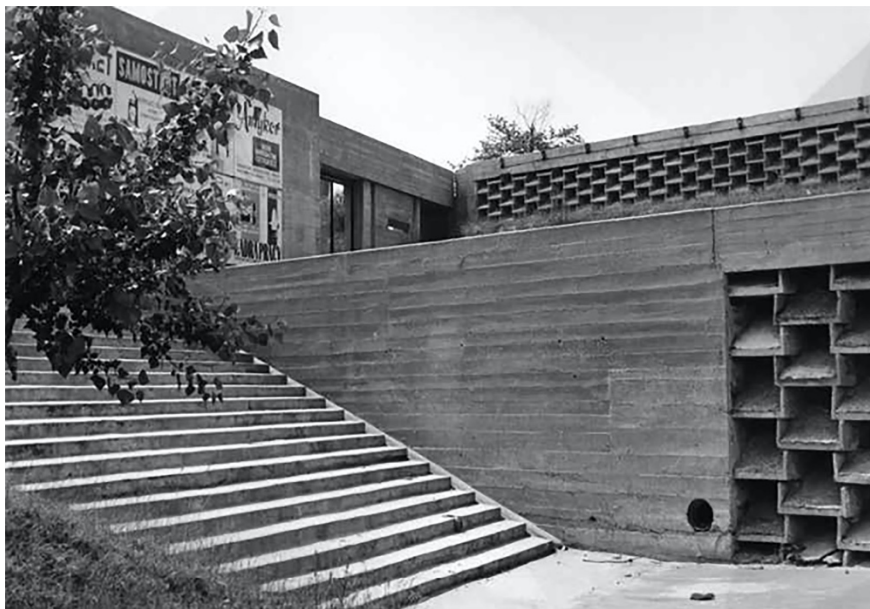
Figure 1. A dedicated type of hollow bricks was designed for retaining walls
