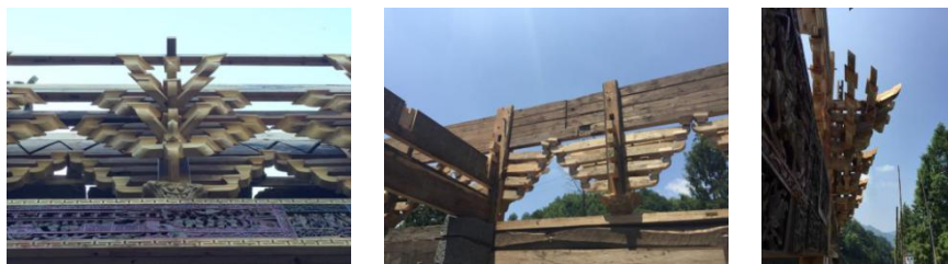
Figure 13. The assembled dougong
