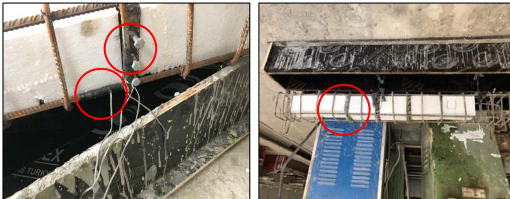
**Figure 6.** Fixing of strain gauges in steel reinforcement.
