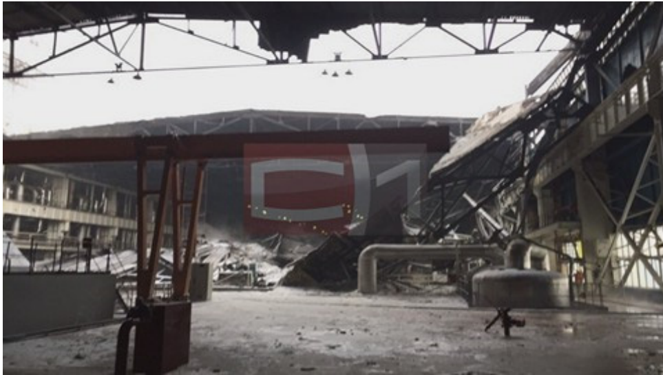
Figure 1. Failed roof of the turbine hall at Surgut power plant unit 4.
