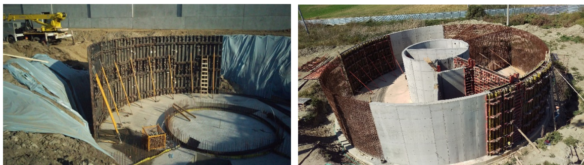
Figure 1. Water tank in Buzau (left) and in Bacau (right) – second phase of casting.
