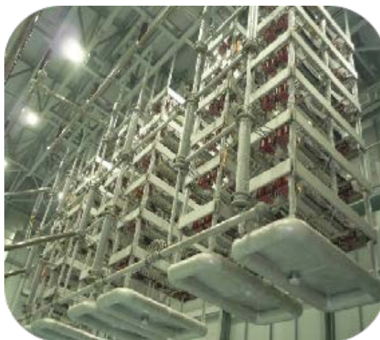
Figure 1. \pm 500\text{kV} HVDC converter valve
