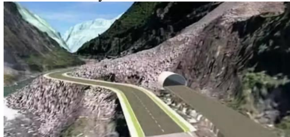
Figure 12. Example of steel corrugated plate temporary passage
