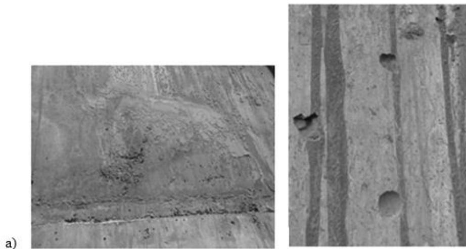
**Figure 1.** Areas with poor compaction of concrete with surface shells
