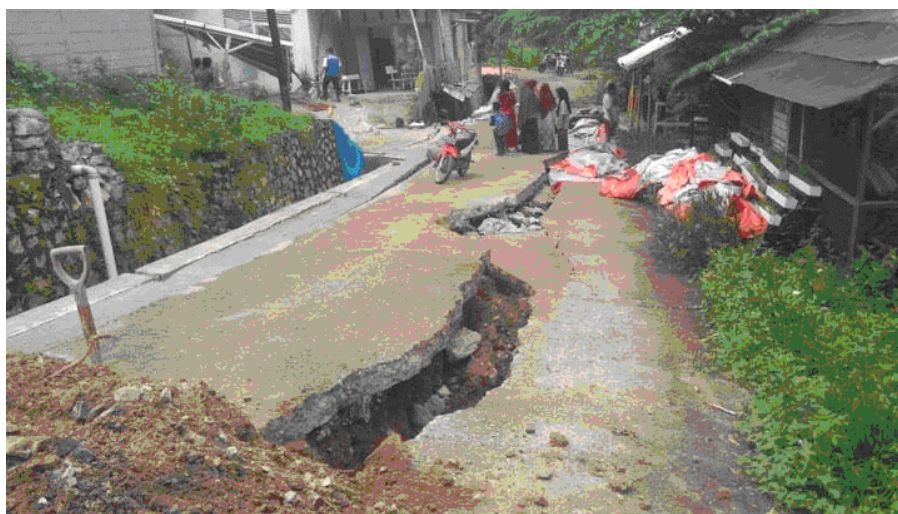
Figure 1. Road damaged by land movement after heavy rains in Santur Village, Sawahlunto, West Sumatra, 2 November 2018. (Photo by BNPB in [6]).
