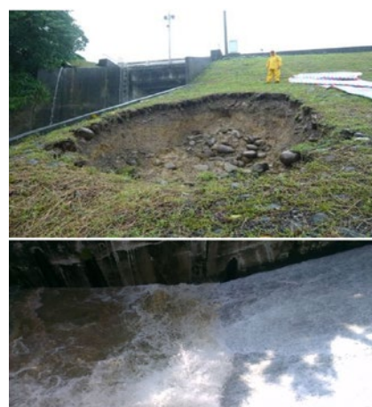
Figure 3. The piping was founded in soil slop beside the spillway after a heavy rainstorm.
