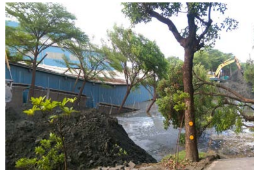
Figure 3. Warehouse subsidence due to subsurface settlement.
