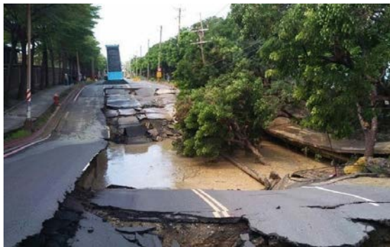
Figure 2. Road subsidence due to subsurface settlement.
