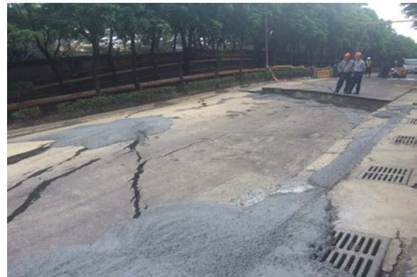
Figure 6. Alligator cracking of the road that occurred due to the land subsidence hazard.
