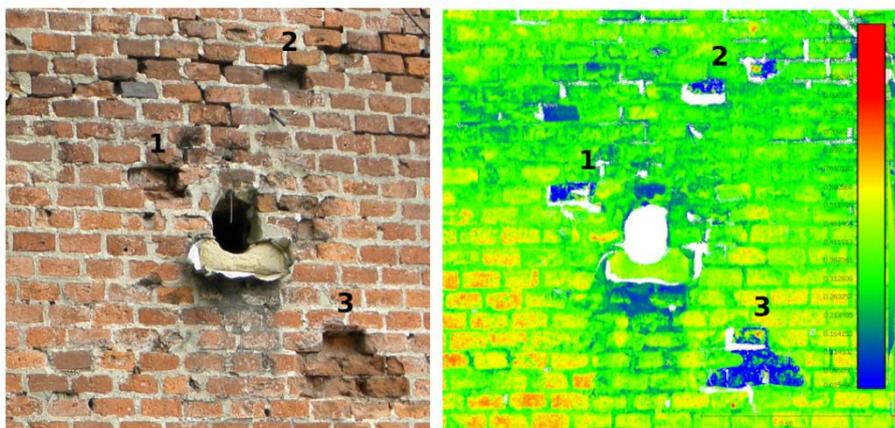
**Figure 5.** Presentation of cavities in the RGB picture and on the point cloud
