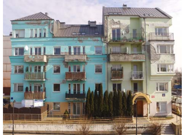
Unit 4 (balconies and tribunes, medium damaged)
