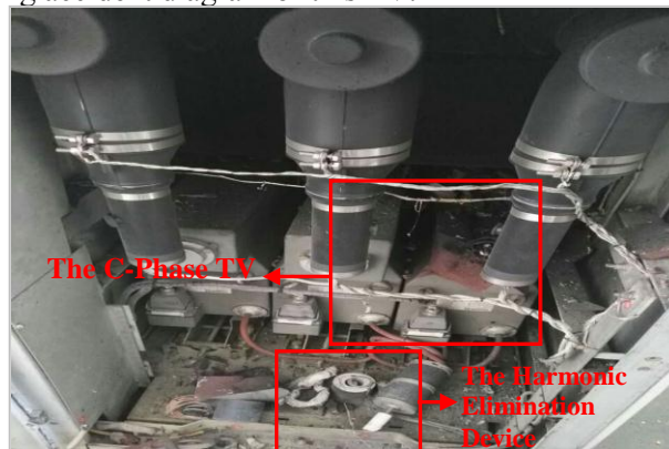
Figure.1 the 35kV Voltage Transformer Burning Accident Diagram
