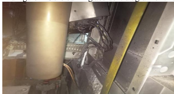
Figure.2 the 10kV Voltage Transformer Burning Accident Diagram
