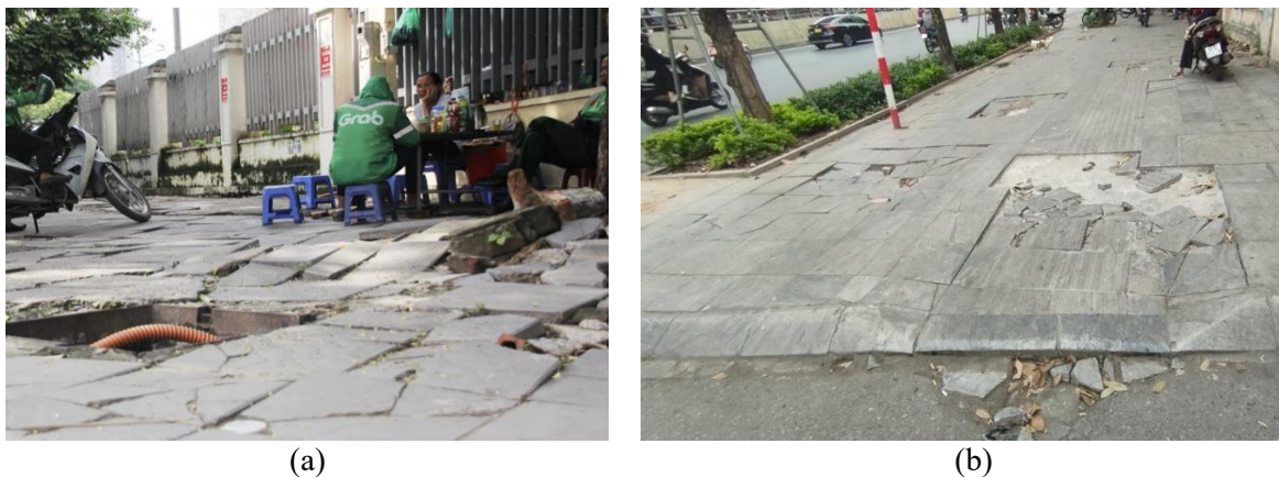
Figure 2. Dilemma reality for Hanoi pavement: (a) Multiple activities on a torn pavement, (b) A popular scene with cracked and broken stone pavements.
