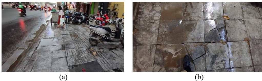
Figure 6. Issues with cracked and broken stone: (a) Always wet and slippery, (b) Water traps.
