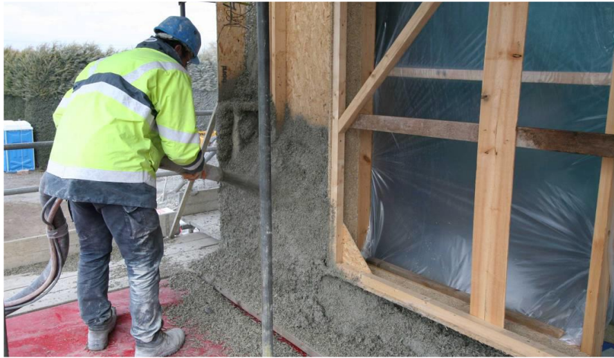
Figure 3. Sprayed hempcrete [37].
