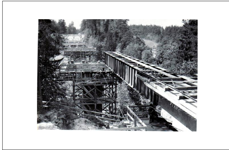
Figure 6. Sliding of span girder section (Latvian Road museum, n.d.)
