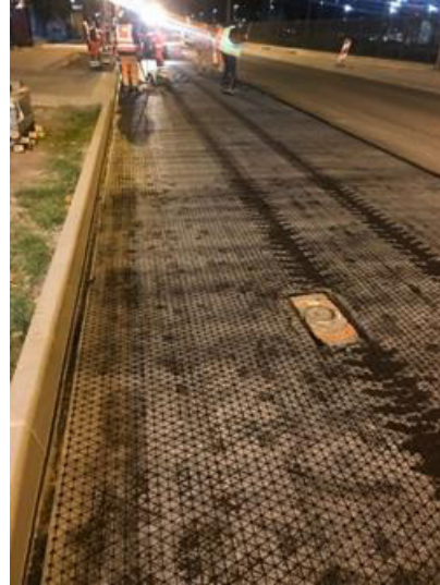
Figure 13. Geocomposite with hexagonal grid installed in place
