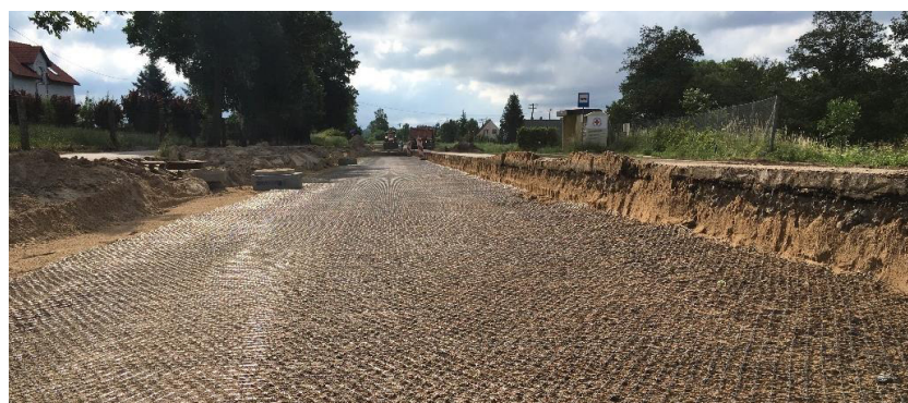
Figure 5. Installation of hexagonal geogrid on road no. 507
