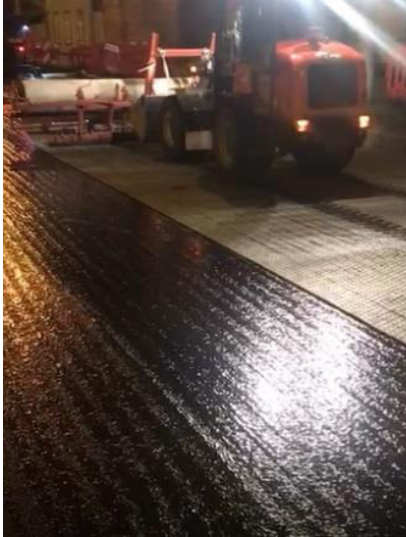
Figure 12. Process of geocomposite installing by the purpose-built asphalt interlayer installation machine
