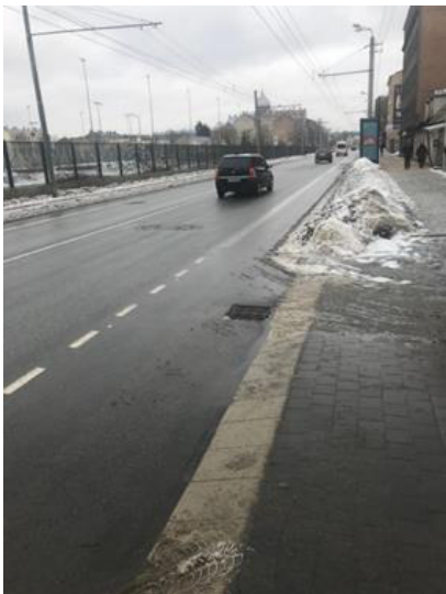
Figure 14. Fully trafficked A. Caka Street. Section strengthened by asphalt overlay with a geocomposite, January 2021
