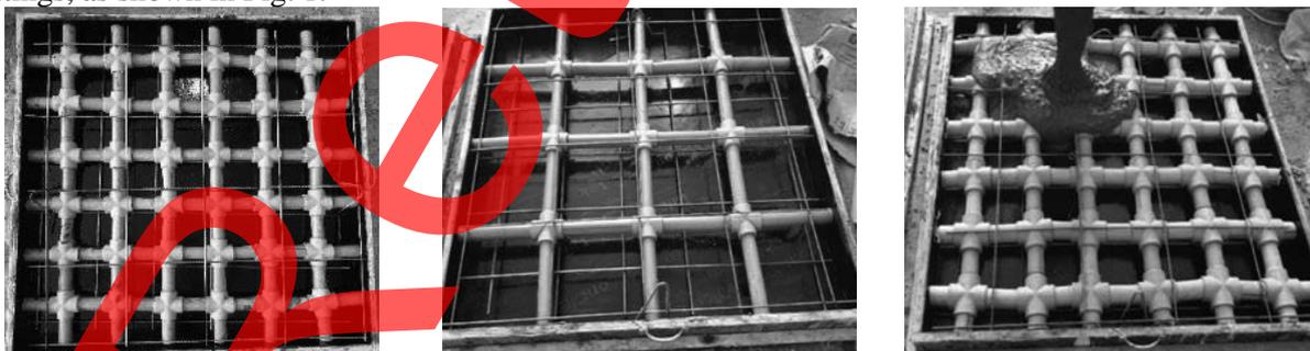
**Figure 1.** Using two-way plastic piping systems in assembling two-way hollow RC slabs.
