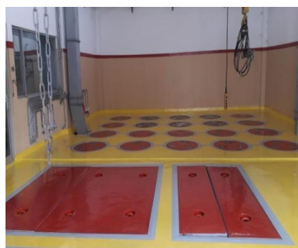
Figure 5. High-level waste storage facility at the RWTC. The red color shapes are the top lid of storage pits. The yellow color is the concrete floor of the facility.
