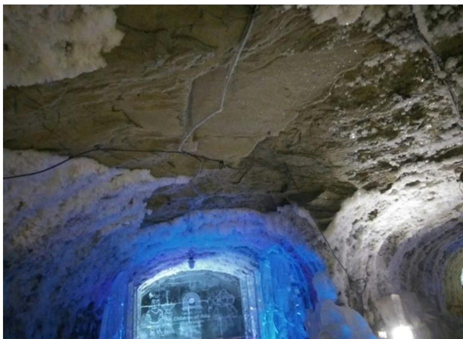
Figure 2. The fall of the roof rocks in the area of the junction of the gallery №1 and the chamber №4 of TKoP.
