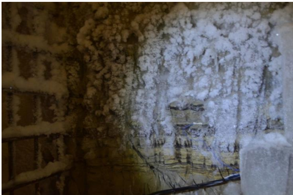
Figure 5. Weathered side of the mine workings of TKoP with an installed temperature sensor.
