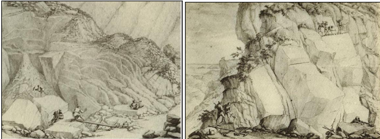
Figure 5. Renaissance cuts: quarrymen used meter-spaced fractures for obtaining slabs (left) or blocks (right).
