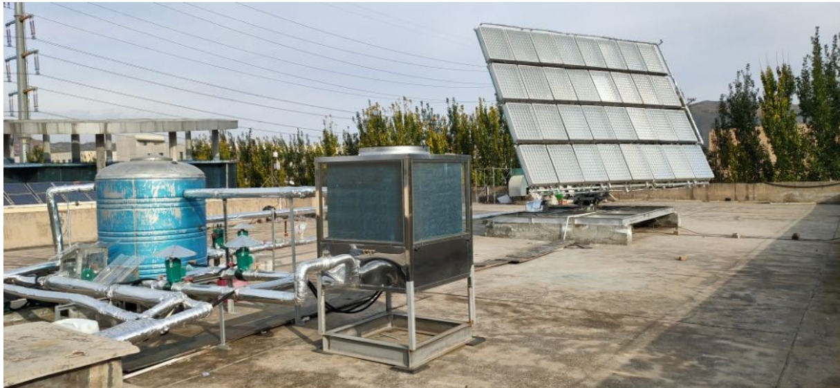
Figure. 1 CPV/T system
