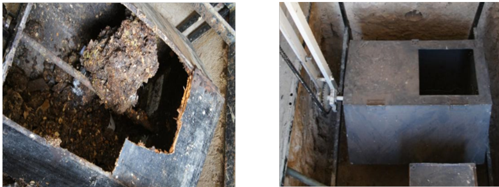
Figure 3. Composting toilet reactor made by wood and metal used in rural Burkina Faso [8].
