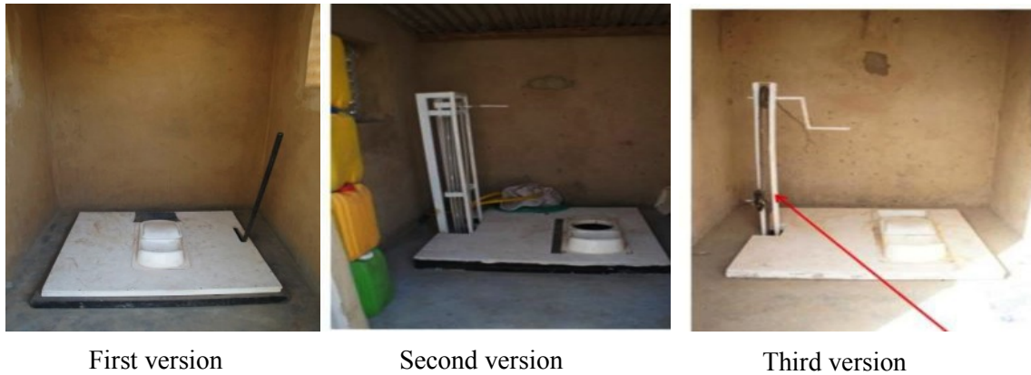
Figure 2. Composting toilet mixing system used in rural Burkina Faso) [8].
