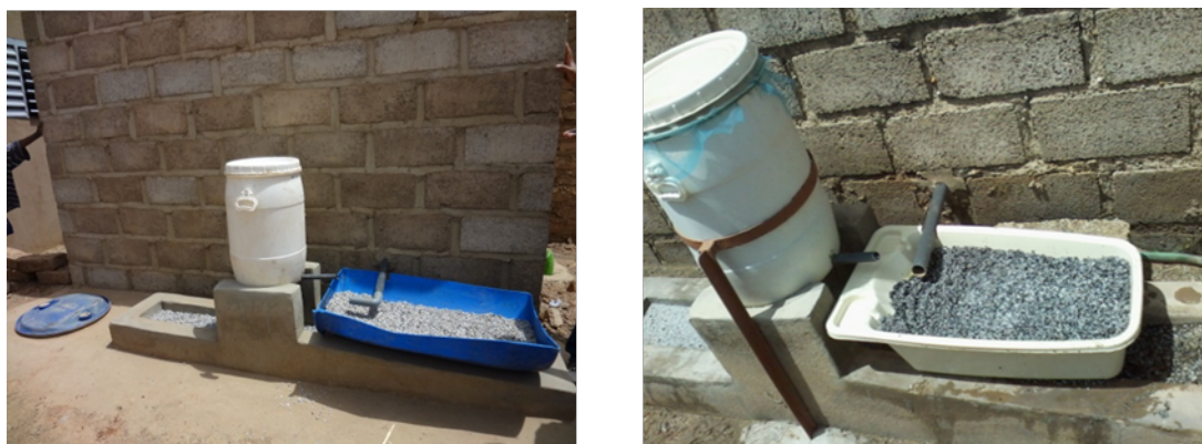
Figure 5. Grey water treatment facility (first and second version) used in rural Burkina Faso.
