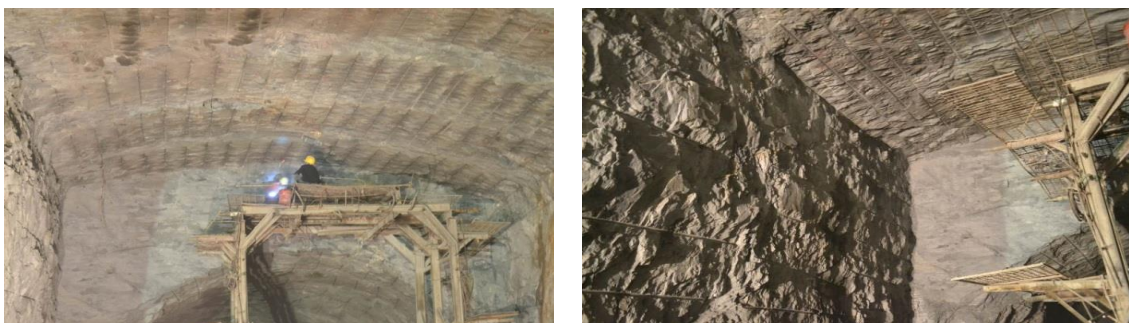
Figure 6. Semi-holes on the rock of tunnel after explosion with cushion pad.
