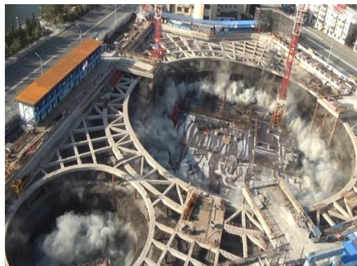
Figure 7. Reinforced concrete support beam blasting demolition photo.
