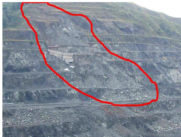
Figure 4. In 2003, Zhujiabao iron open-pit of Panzhihua Steel Group (Sichuan province), blasting induced slope slide.
