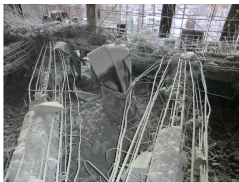
Figure 8. Photo of reinforced concrete beam after blasting.
