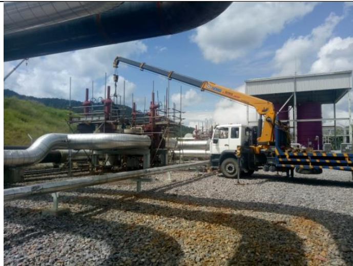
Figure 6. Replacement suction strainer.
