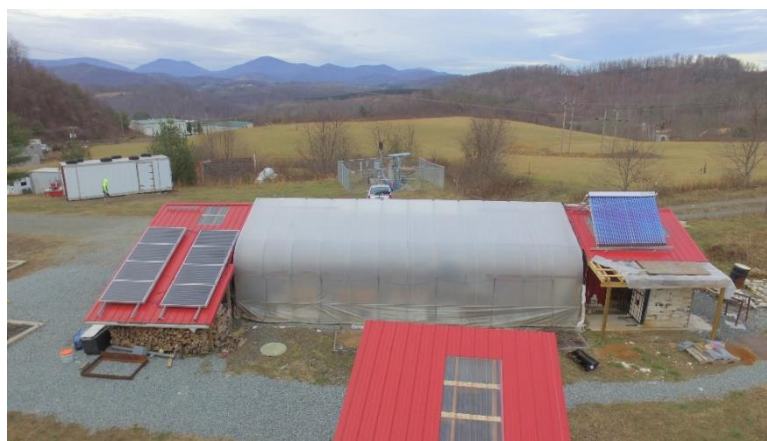
Figure 3. Photovoltaic (left) and Solar thermal (right) installed at Nexus.
