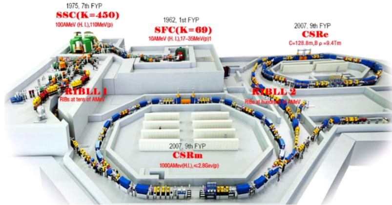
**Figure 1.** Layout of Heavy Ion Accelerator Research Facility in Lanzhou (HIRFL).
