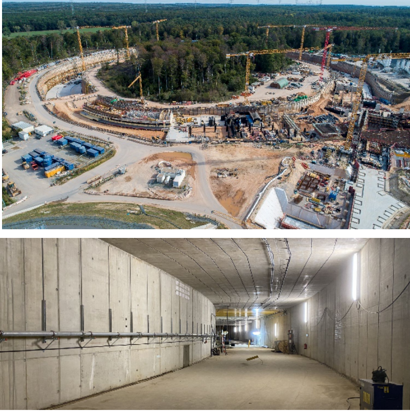
Figure 7. Top: SIS100 open pit tunnel construction including the shell construction of the crossing building (right) and the connecting tunnel to SIS18. Bottom: completed section of the SIS100 accelerator tunnel from the inside.
