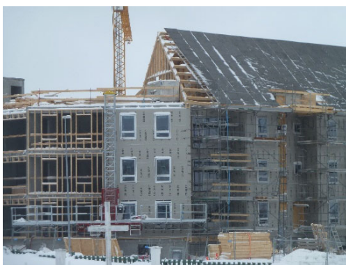
Figure 3. Multi-storey building with wood-based facades before and after installing wind barrier, and wood-based roof construction with roofing felt.
