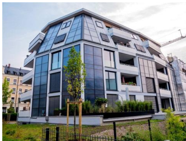
Figure1. Apartment building designed as a solar house with a modern, futuristic-looking solar architecture. A total of 317 square meters of solar collectors were integrated into the east facade and the south-facing gable side.
