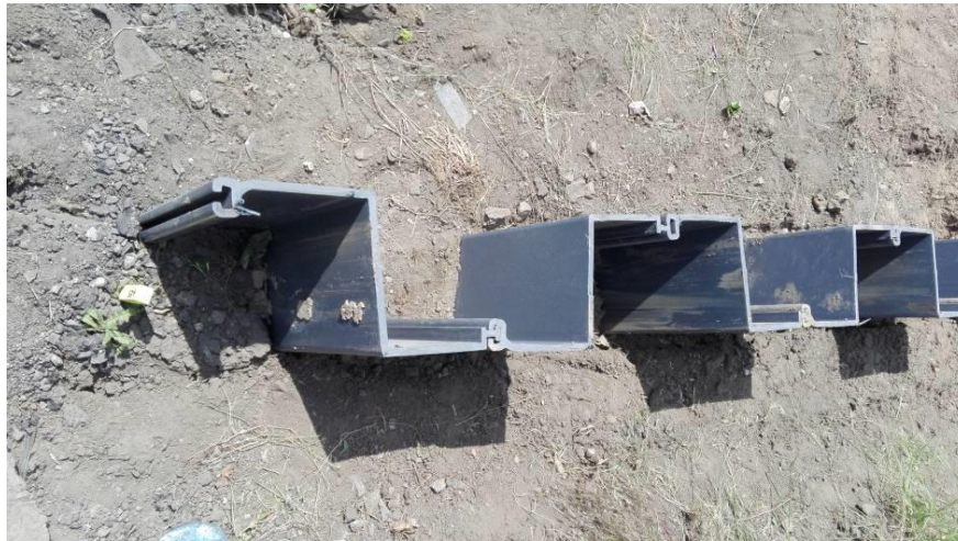
Figure 1. Vinyl sheet piles with interlocks after driving.
