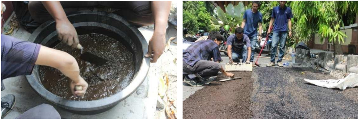
Figure 1. The Implementation of Slurry Seal
