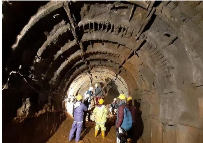
**Figure 4.** Supports provided in the HRT of Super Madi HEP (4.2m diameter tunnel).
