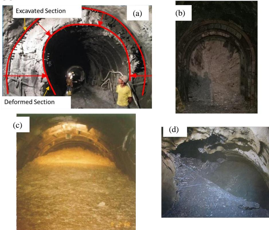
**Figure 1.** Tunnelling Problems in the Himalayas (a) Squeezing in Chameliya HRT, (b) Face collapse in Sanjen HRT, (c) Water inflow in Modi HRT and (d) Roof Collapse in Kaligandaki A HRT [2],[4],[6].
