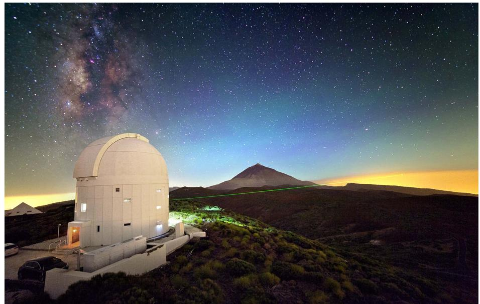
**Figure 12.** The OGS (Optical Ground Station) established on the island of Tenerife by the European Space Agency ESA. This telescope is used in our tests of long-distance quantum communication between the Canary Islands of Tenerife and La Palma which are separated by about 150 km. The laser beam shown is an alignment laser going over to La Palma. At the end of the laser line, one sees a bright spot, which is another alignment laser pointing from La Palma to Tenerife. Photo: Daniel Padrón.
