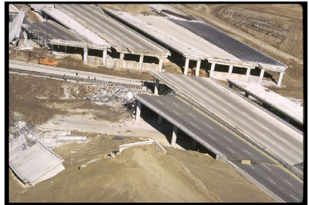
Figure 3. Unseated spans in the 210/5 Interchange during the 1971 San Fernando earthquake (NISEE Collection).
