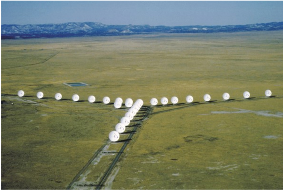
Figure 1. Aerial photograph of the VLA in its most compact “D” configuration, with maximum baseline 1.0 km. The array can be reconfigured by moving the antennas to more distant pads via the rail lines visible in the photograph. (A color version of this figure is available in the online journal.)
