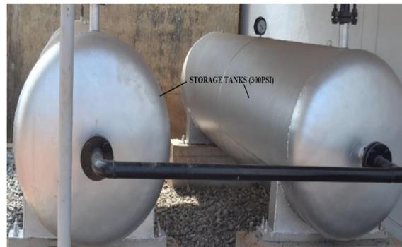
**Figure 1.** Photographic view of storage tanks
