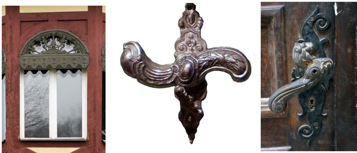
Figure 7. Cast iron elements of the elevation of the building; on the left side: lambrequin in form resembling the fabric; in the middle: window-handle; on the right side: door-handle in a shape of a lion.
