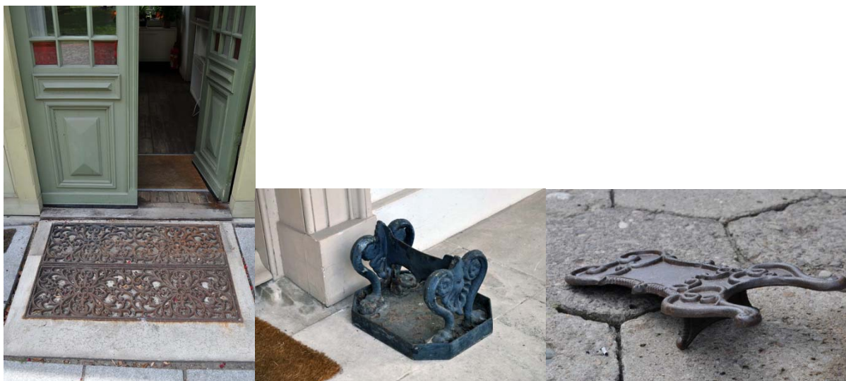
Figure 5. Cast iron items related to the shoes. On the left side: flat wiper with floral motifs; in the middle: the scraper with decoration on both sides and a tray for the dirt; on the right side: the puller used to remove the boots in a shape of angled plate with decorations and an indentation for the back of the shoe
