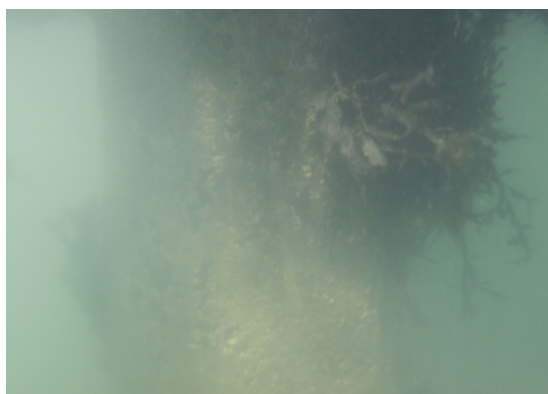
Figure 5. Marine growth affected pile.
