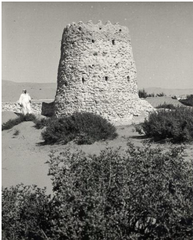
Figure 7: Hayla Tower in undated historic photograph (circa mid-20 th century). Source: CDR.
